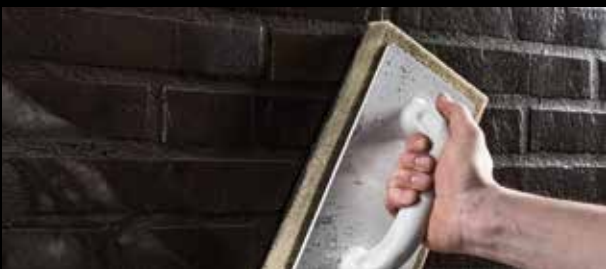
The excess grout is washed off diagonally using a plaster float with a sponge or foam pad.
