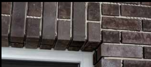
Window lintel perfectly replicated with angles.
