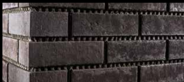
The finished surface. Grouting can be done after the appropriate drying time.
