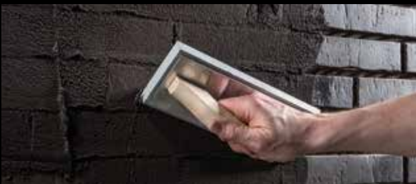
With the slurry method, the joints are filled diagonally with the grouting or plaster float. Walls should be worked from top to bottom.
