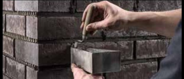
The vertical joints can be finished more easily with a smaller pointing trowel.
