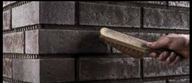
Sweeping out the joint gives it a corresponding structure.
