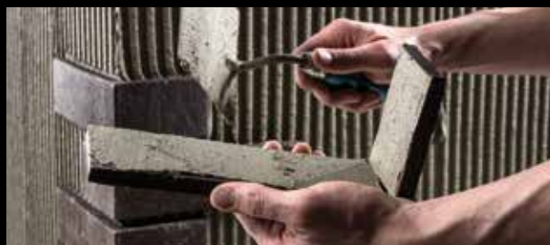
The corner angles are worked using the floating-buttering method.
