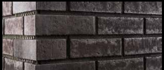
The finished joint pattern. Full masonry stretches are grouted at one go.
