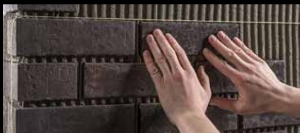
Use a string to plumb the clinker area. The clinker slips are pressed into the adhesive bed.
